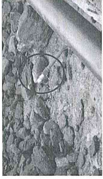
Fixed type DS system at Coal Yard
